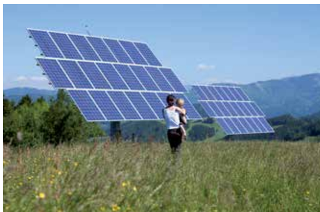
Photovoltaikanlage. Fotos: BIO AUSTRIA
